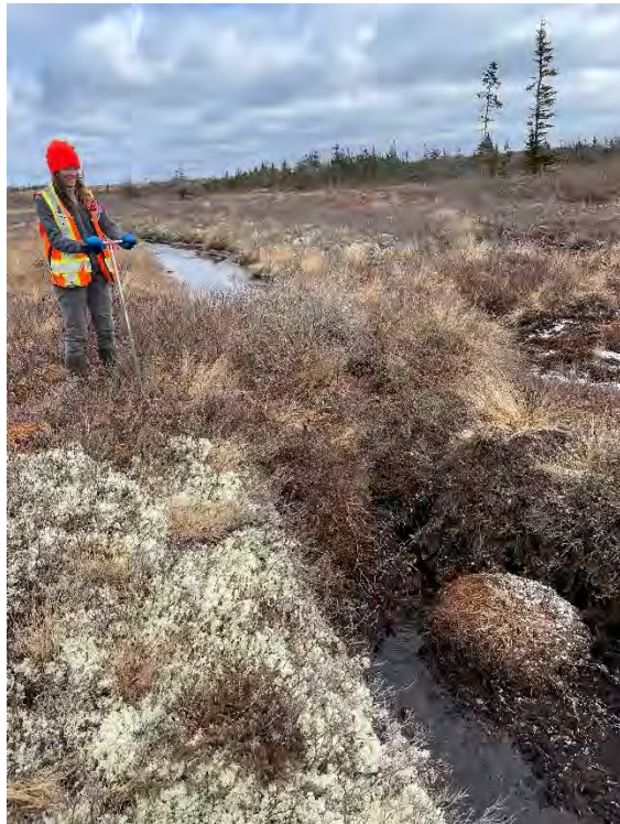
Photo 9: Example of eroded ditch block of main exterior ditch. Water levels vary by >1 m on either side of the block.
